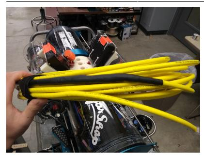
Slide the large heat shrink over the splice and shrink it down with the heat gun at 90 degrees Celsius. Make sure it is completely shrunk down and your done!
